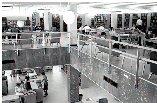
Max Chambers Library, 1957, today the Communications Building
